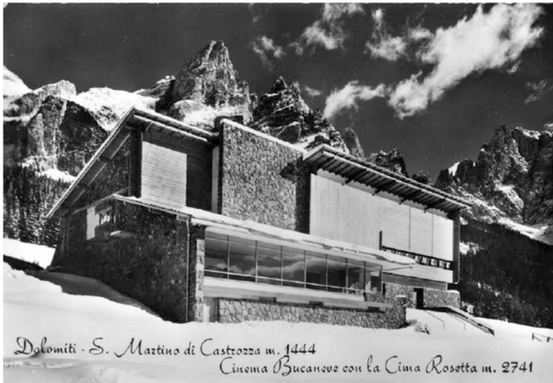
Fig. 3. Cinema Bucaneve (arch. Toffol)
